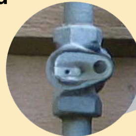
Closed gas meter valve
